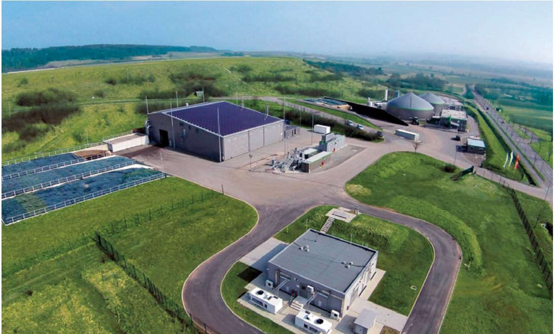
Abb. 9.7 Biogasanlage Allendorf (Eder) (Foto: Viessmann)
