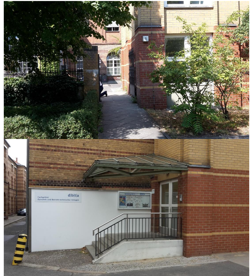
Instructions for getting to the KWT-N building (secretariat and office Prof. Repke)
