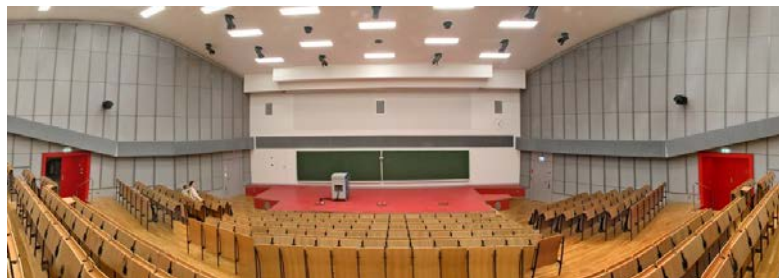
Figure 1.1: Auditorium H 104 at TU Berlin. Multichannel system of 832 separate channels for wave field synthesis. More than 2700 loudspeaker arranged in 10 cm distance on ear-level around the audience.
